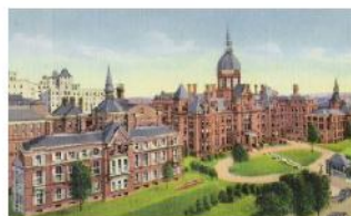
John Hopkins Hospital de Baltimore, USA
